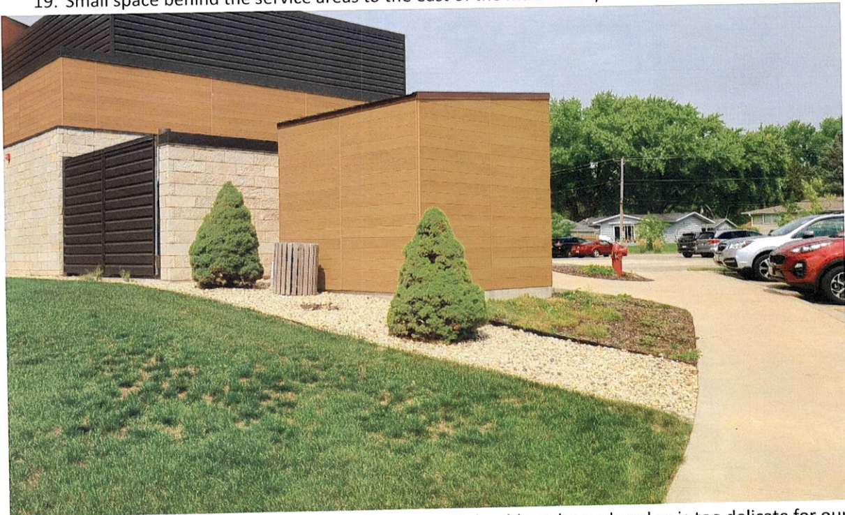
19. Small space behind the service areas to the east of the main library.
